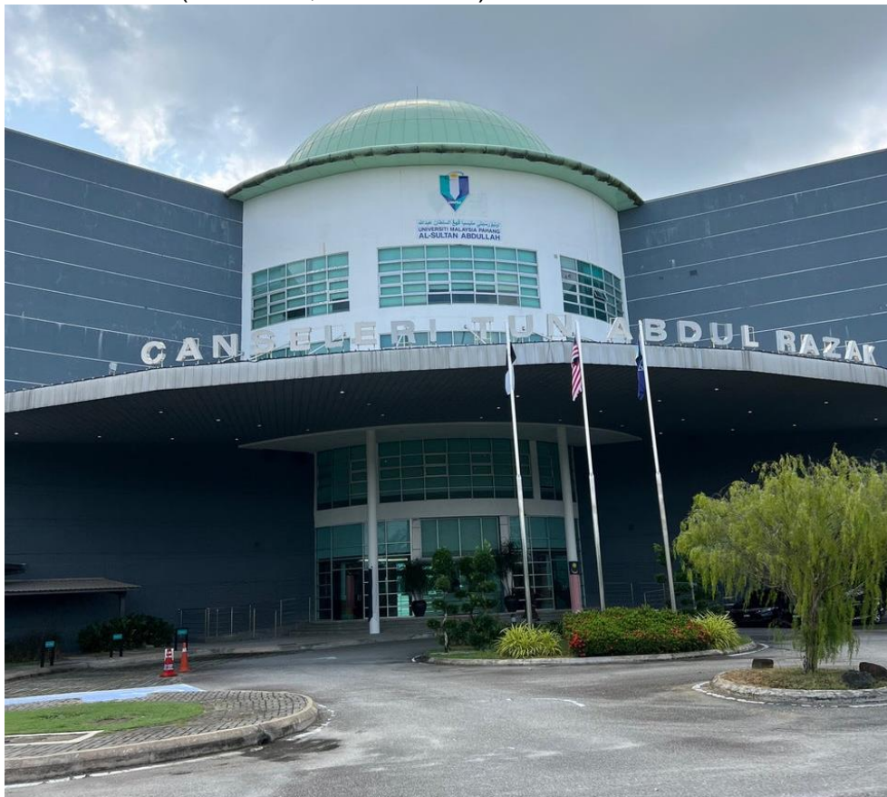
CTAR UMPSA Pekan Charging Station
