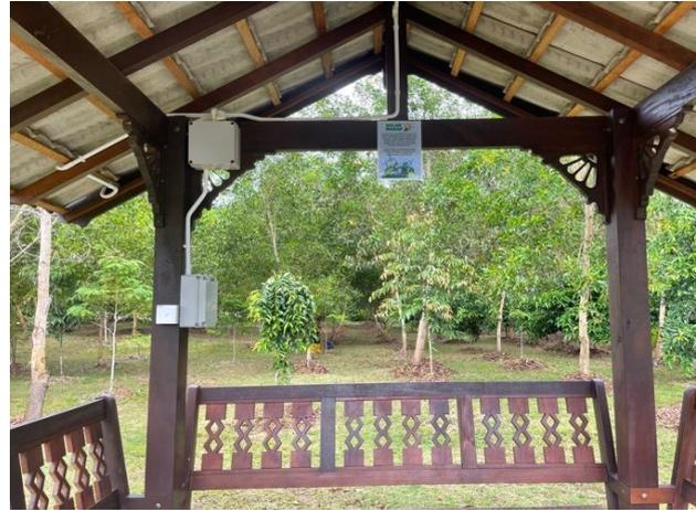
There are 20 waqf huts inside UMP Pekan & UMP Gambang equipped with solar systems. This 100W solar produces electricity for lights, and phone chargers. There is also a Power Delivery Charger for laptop charging and other electronic devices ranging from 5V - 12V. For phone charging, there are 2 options for charging mechanism:
