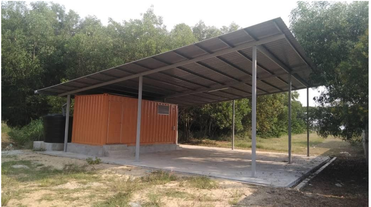
Compost & Recycle Centre, UMP Pekan
