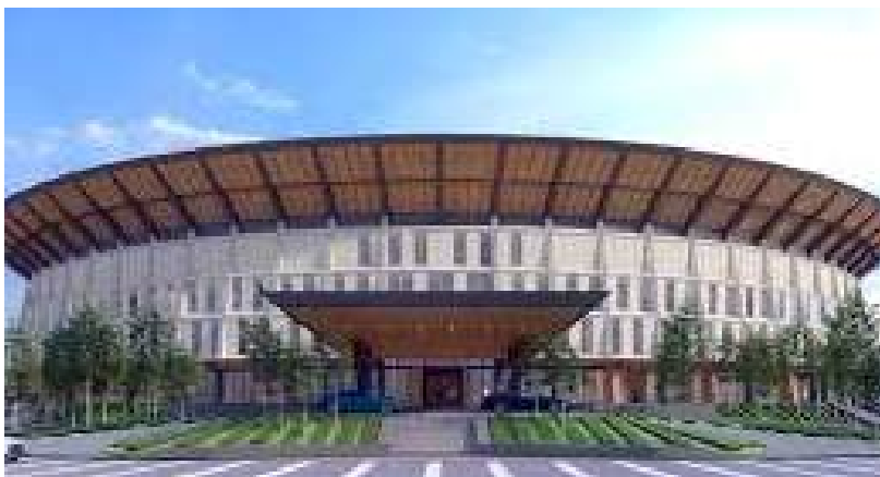
Convocation Hall UMPSA. Expected completion 2026
